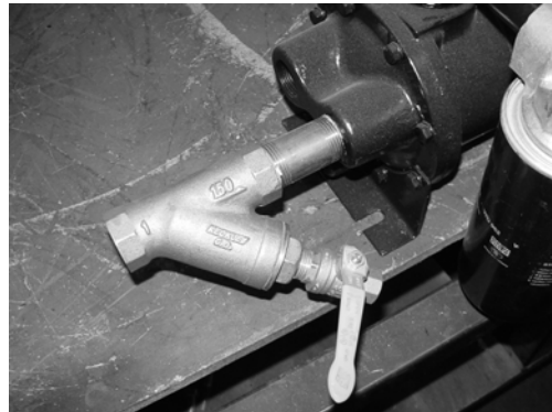
Figure 4 Wye-strainer installed, with cleanout valve
