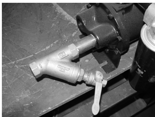
Figure 4 Wye-strainer installed, with cleanout valve.
