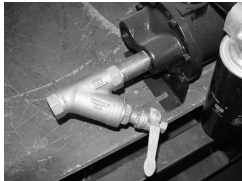
Figure 3 Wye-strainer installed, with cleanout valve.
