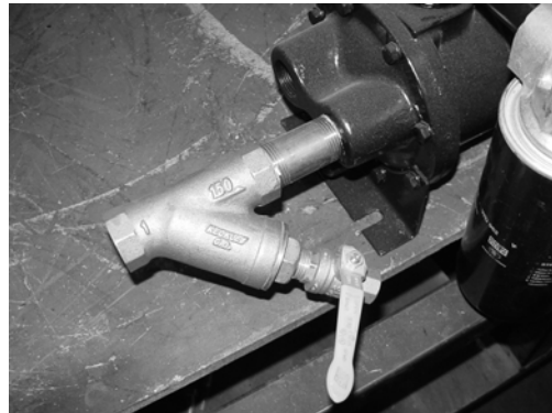
Figure 5 Wye-strainer installed, with cleanout valve.
