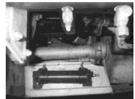
Cooler mounted on the side of a pump compartment with the cooler body sloping toward the drain for better drainage.
