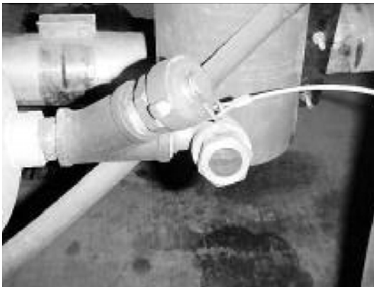
Figure 12 90° Elbow on a sight glass for better visibility
