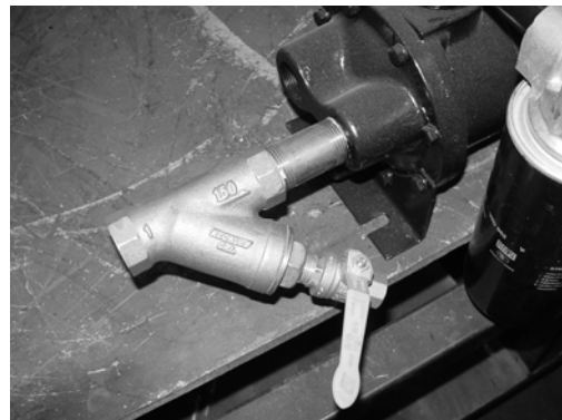
Figure 18 Wye-strainer installed, with cleanout valve.
