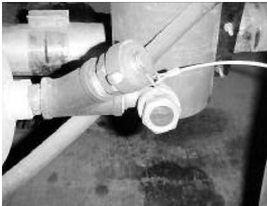
90° Elbow on a sight glass for better visibility
